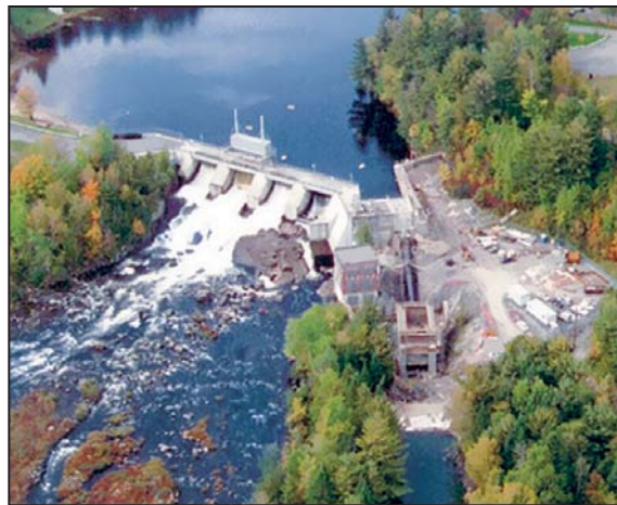
Figure 6: Small Hydro System.
