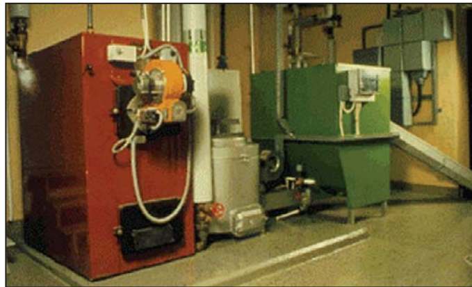
Figure 8: Biomass Heating System
